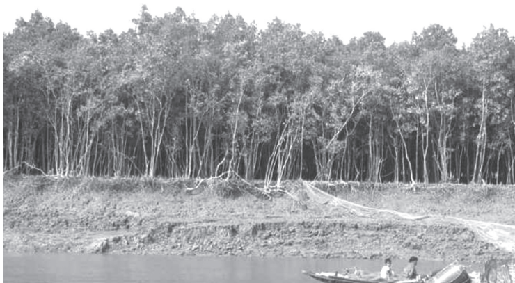
Pic No: 4. Bank erosion of Matla River. Source: Self Click
